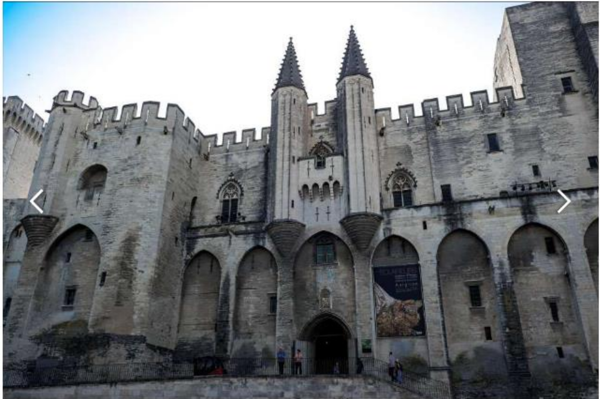
Photo: Mark Sissons, Special To The Chronicle
