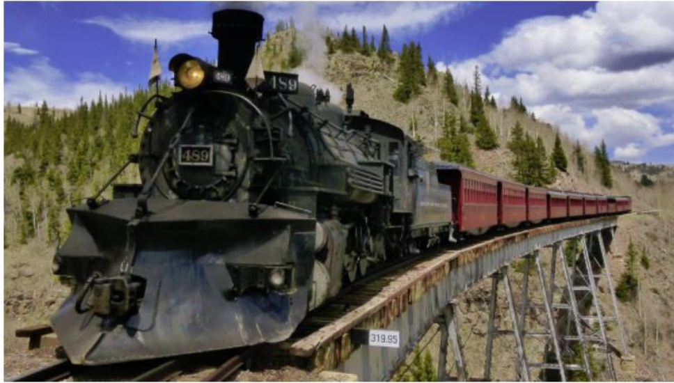
The Cumbres & Toltec Scenic Railroad runs 64 miles between Antonito, Colo., and Chama, N.M. Photo Credit: Rich Grant, Cumbres & Toltec Scenic Railroad
