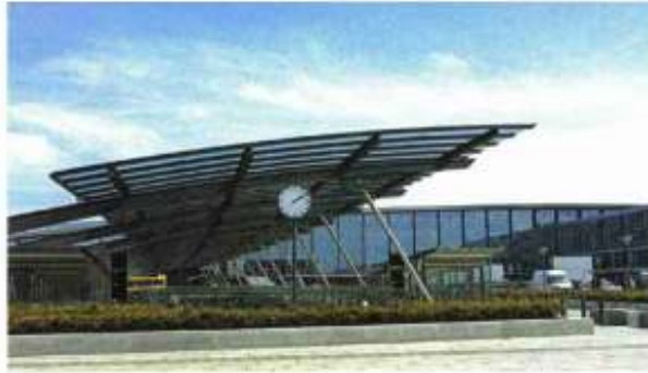
The basic shape of Terminal 3 was inspired by an aircraft wing. Designed by the Vilhelm Lauritzen firm of architects and made of glass, steel, aluminum, and granite, T3 was built in 1998.
